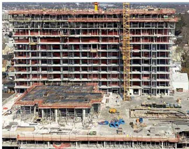
Fig. 2.9.12: Formwork and reinforcing bars for the tower in the background are being staged on top of the base structure in the foreground. (Image courtesy of CKC Structural Engineers.)
