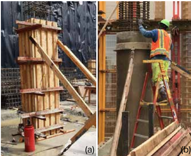
Fig. 2.6.17: Examples of concrete column forms: (a) rectangular; and (b) round. (Images courtesy of Conco.)
