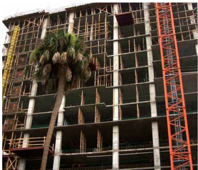
Fig 2.6.38: This project included an upper-level floor with a large dead load. Seven levels of reshores were needed to support the placed concrete. The reshores delayed finish trades in the affected levels and extended the overall construction schedule until sufficient concrete strength was attained on the freshly placed level to allow removal of shoring. (Image courtesy of Mary Bordner Tanck.)
