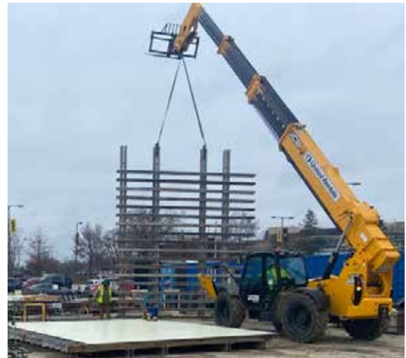
Fig. 2.6.5: Workers engage in the make-up of a large gang form. Larger panels require onsite labor, area, time and hoisting to support the make-up. Further, they are too large to assemble off site and truck to/from the site. A similar disassembly process is required upon completion of use. (Image courtesy of Ceco Concrete Construction.)
