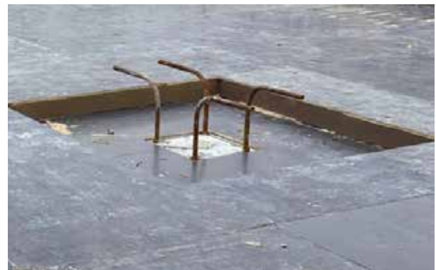
Fig. 2.6.34: A drop panel has been formed and is awaiting reinforcement installation. Better constructability is achieved using shear studs in lieu of a drop panel (refer to Section 2.7(h)). (Image courtesy of Ceco Concrete Construction.)
