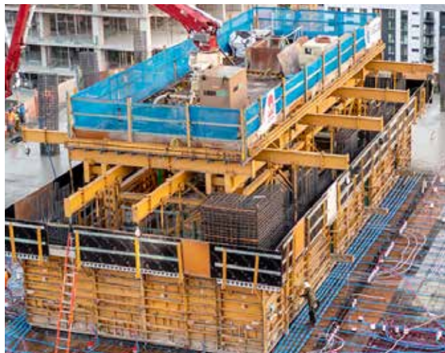
Fig. 2.9.5: A self-climbing formwork system topped by a work/storage platform and a placing boom. The entire system is lifted by hydraulic jacks from embeds in previously poured walls below the system. (Image courtesy of The Conco Companies.)
