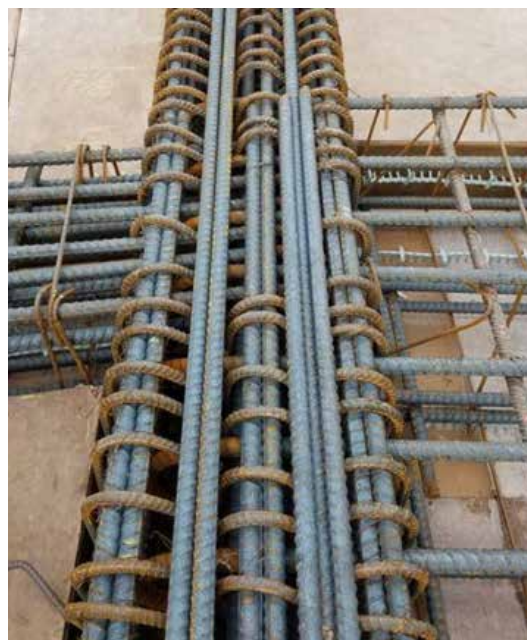
Fig. 2.2.1: Designers must be aware of the need to place and consolidated concrete. (Image courtesy of Ceko Concrete Construction.)
