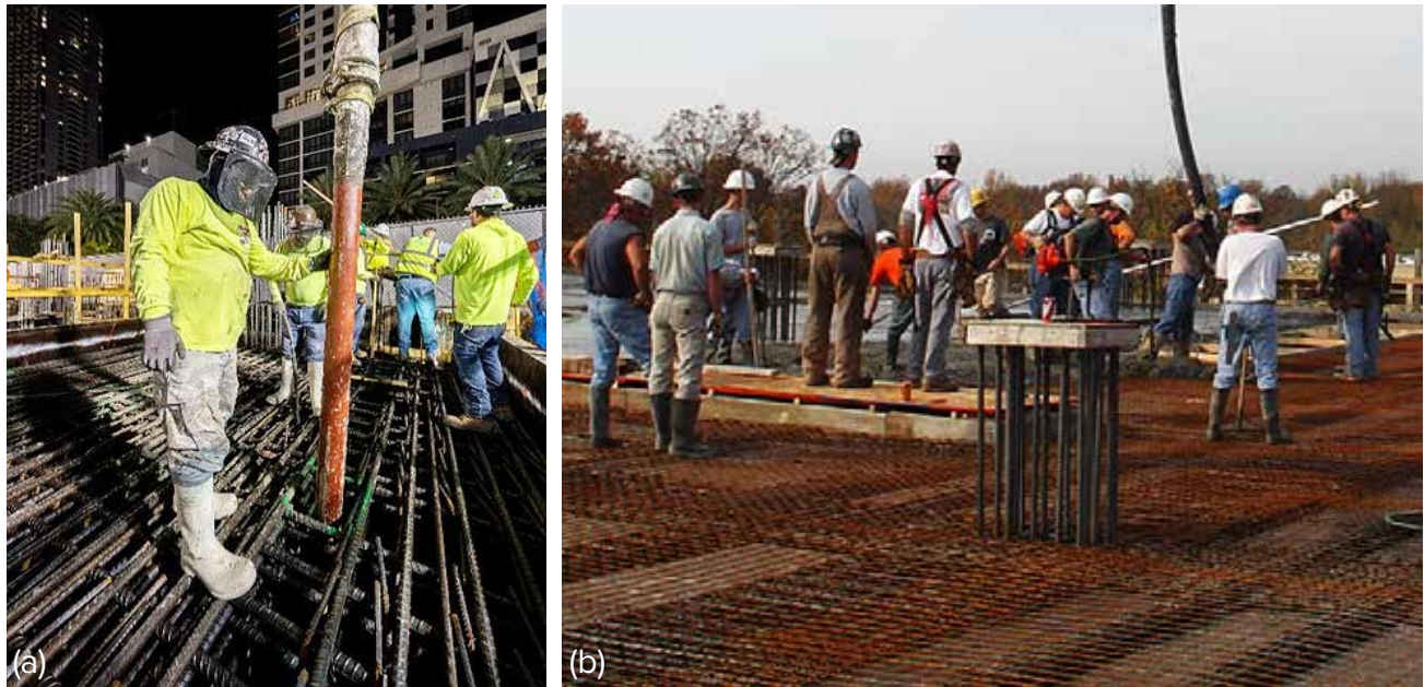
Fig. 2.7.15: Crews must walk on the reinforcing in thick slabs and foundation mats during concrete placements. Safe footing can be provided using: (a) grid of closely spaced reinforcing bars; or (b) welded-wire reinforcing placed on top of larger, more widely spaced bars. (Images courtesy of Ceco Concrete Construction.)
