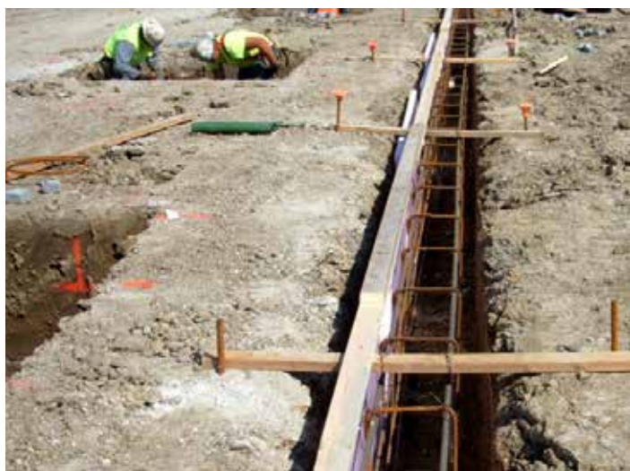
Fig. 2.12.2: Photos of continuous footings that have been prepared for bank pours. (Image courtesy of Ceco Concrete Construction.)
