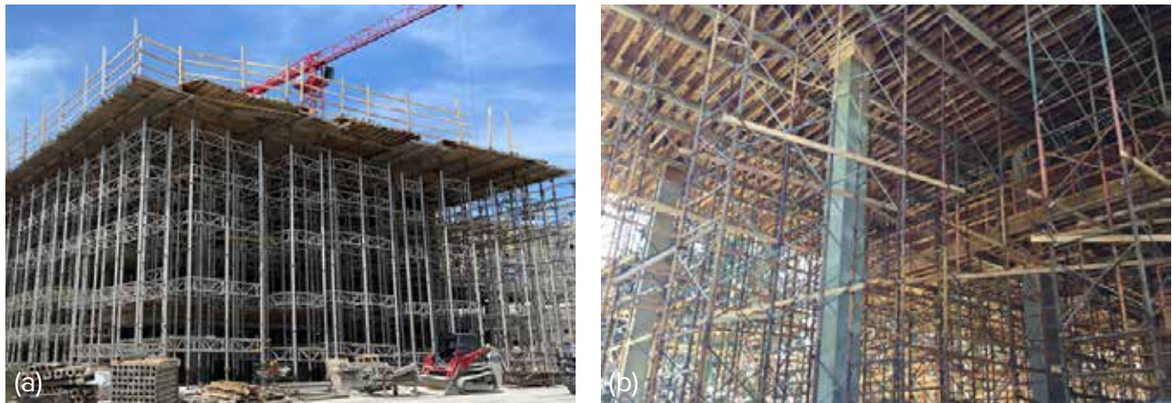
Fig. 2.6.26: Examples of high shoring. ((a) Image courtesy of Ceko Concrete Construction. (b) Image courtesy of Conco.)
