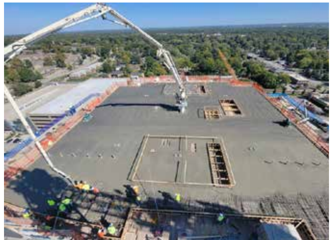
Fig. 2.9.8: A placing boom coupled to a standpipe accommodated through a blockout in the floor slab. In this photo, the placing boom is mounted on a pedestal and anchored to the floor slab(s). These construction loads in the floor slab should be considered prior to installation. (Image courtesy of Ceko Concrete Construction.)
