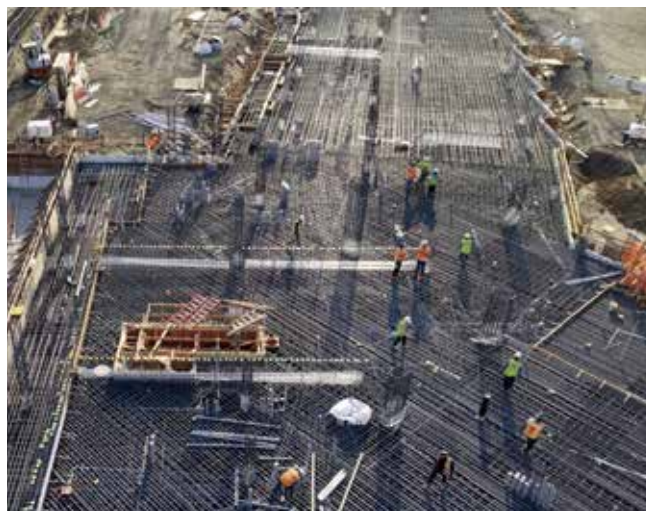
Fig. 2.12.6: A “mat slab” foundation. (Image courtesy of Related.)
