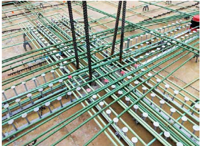
Fig. 2.7.48: Stud rails or double-headed studs can help designers avoid the need for drop panels. (Image courtesy of Amsysco.)
