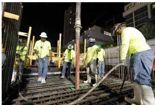
Fig. 2.7.2: Early communication between the contractor and designer resulted in the development of preplanned openings in the reinforcing mat for insertion of the concrete pump hose. (Image courtesy of Ceko Concrete Construction.)
