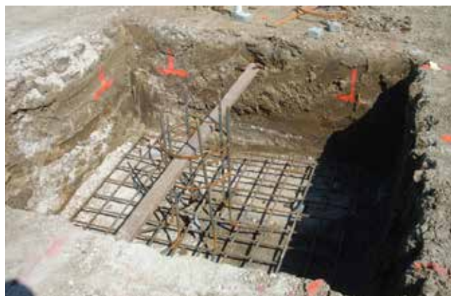
Fig. 2.12.1: Photo of excavation and reinforcement for an isolated spread footing with soil-formed sides. The concrete placement is commonly termed a “bank pour.” (Image courtesy of Ceco Concrete Construction.)
