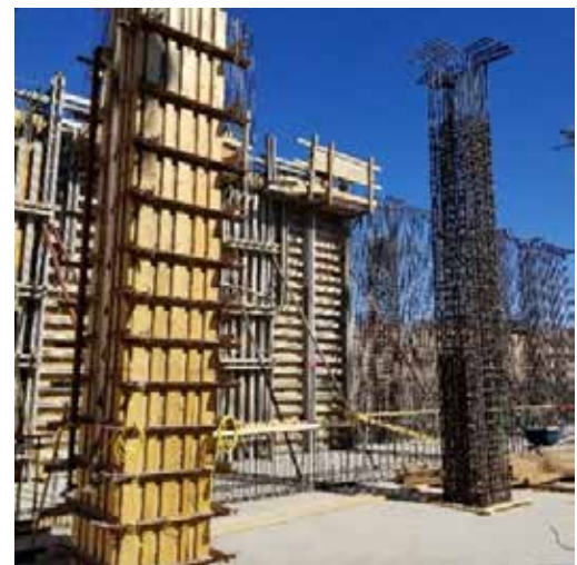
Fig. 2.6.2: When possible, use the same column size and geometry over the full area of the building and maintain column sizes over at least 10 floors. (Image courtesy of Ceco Concrete Construction.)
