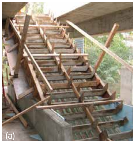
Fig. 2.6.25: Construction of concrete stairs: (a) cast-in-place concrete; and (b) precast concrete. (Image courtesy of Ceco Concrete Construction.)
