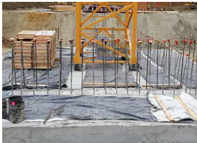
Fig. 2.9.2: A tower crane foundation. (Image courtesy of The Conco Companies.)
