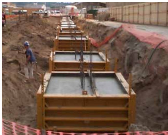
Fig. 2.6.24: While designing footings to have matching depth and alignment aids in constructability, even greater constructability may be achieved by replacing closely spaced footings with a continuous footing. (Image courtesy of Ceco Concrete Construction.)
