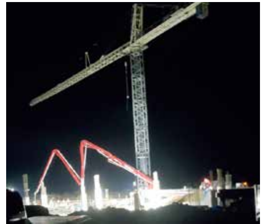
Fig. 2.9.15: Examples of night placements. (Images courtesy of Ceko Concrete Construction.)
