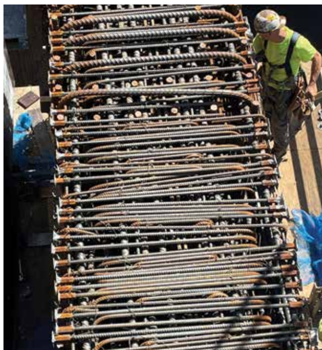
Fig. 2.7.1: The reinforcement in this member approached 800 lb/yd 3 and clearly presented a constructability challenge. (Image from “ Reinforcement Congestion in Cast-in-Place Concrete ,” Concrete International, December 2022 ( ascconline.org ).)
