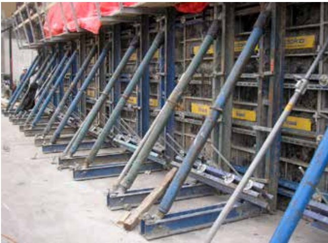
Fig. 2.12.9: One-sided wall form with base anchors and adjustable braces required to withstand the pour pressure without formwork tie rods. (Image courtesy of Ceco Concrete Construction.)
