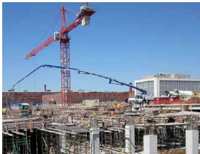
Fig. 2.9.10: A boom pump and two concrete trucks delivering concrete from a position on top of a previously constructed deck section. (Image courtesy of Ceco Concrete Construction.)
