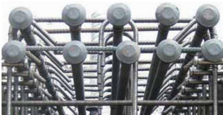
Fig. 2.7.32: Headed reinforcement can help avoid congestion and ensure adequate embedment to develop bars. (Detail source: STRUCTURE Magazine, May 2011, "Tips for Designing Constructible Concrete Structures, Part 2." Image courtesy of Headed Reinforcement Corp.)
