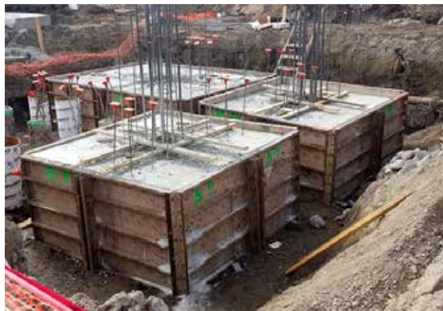
Fig. 2.12.5: An example of a lost opportunity to improve constructability by using spot footings in lieu of a continuous or mat footing. (Image courtesy of Ceko Concrete Construction.)
