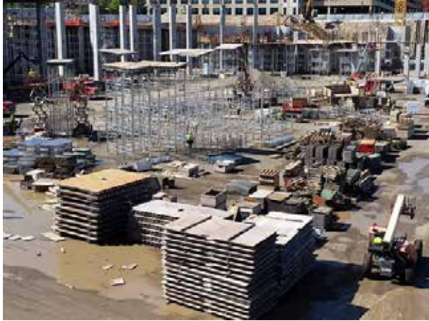
Fig. 2.6.13: A project “boneyard” of idle formwork. (Image courtesy of Ceco Concrete Construction.)
