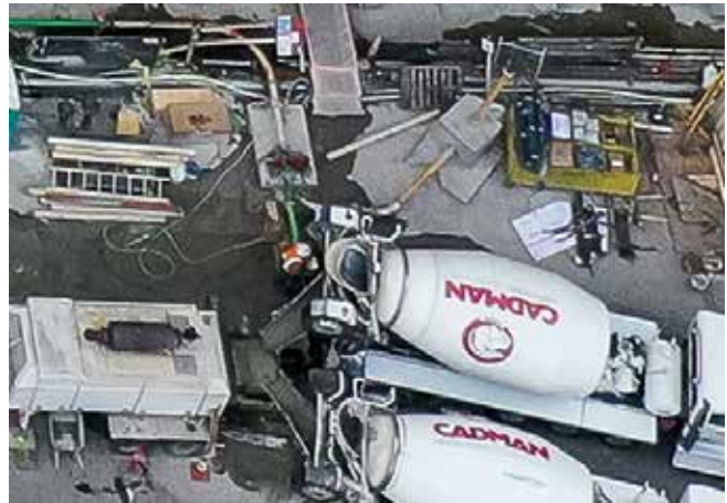
Fig. 2.9.7: A trailer pump with slick line. Access for two concrete trucks remains critical for concrete placing productivity. (Image courtesy of Ceko Concrete Construction.)
