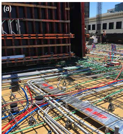
Fig. 2.7.40: Non-structural embeds can conflict with reinforcing bars and strands: (a) sleeves, conduit, and ducts can create major conflicts within elevated slabs; and (b) a 3-D model with all embedded structural and non-structural systems in a floor structure can help the design team avoid conflicts that will ultimately add cost to the project owner. (Images courtesy of CKC.)
