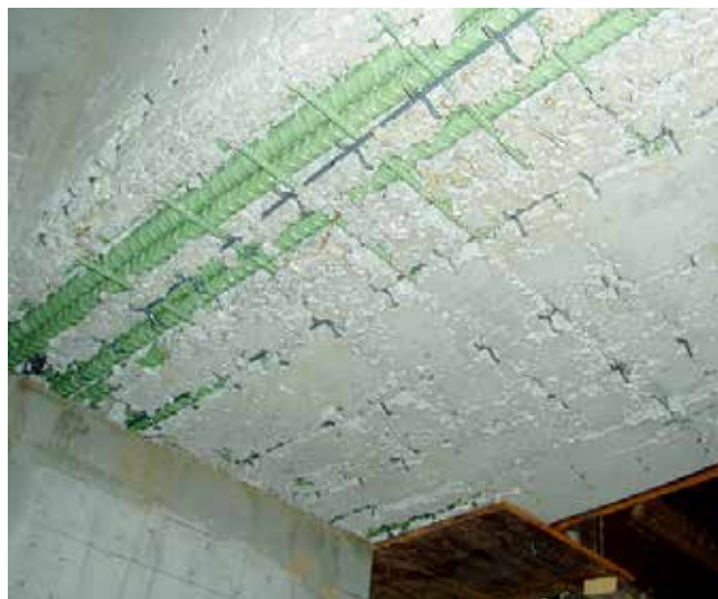
Fig. 2.8.6: An example of a beam with large coarse aggregate, inadequate cover, and spacing between bars. (Image courtesy of Ceco Concrete Construction.)
