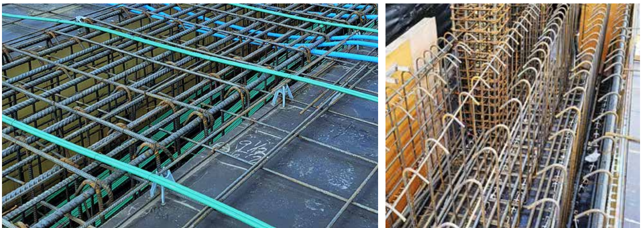
Fig. 2.7.24: Wide beams with multi-leg stirrups, open to the top. The beam cage can be closed using a separate top cap. (Image courtesy of Conco.)
