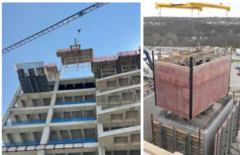
Fig. 2.6.8: Movement of panelized formwork systems requires crane time, capacity, reach and clear area below the load when beyond the building perimeter: (a) lifting a perimeter table panel to the next level; and (b) hoisting an interior core wall gang form. (Images courtesy of Ceko Concrete Construction.)
