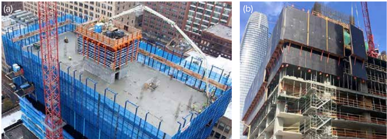
Fig. 2.9.13: Examples of protective screening systems: (a) an aerial view of a cocoon during a concrete pour (image courtesy of Ceco Concrete Construction); and (b) a street view of a cocoon segment during installation (image courtesy of Related).
