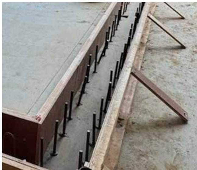
Fig. 2.8.5: Construction of a curb. Dowels have been installed by drilling and setting in adhesive anchors, and the formwork has been installed. (Image courtesy of Hensel Phelps.)
