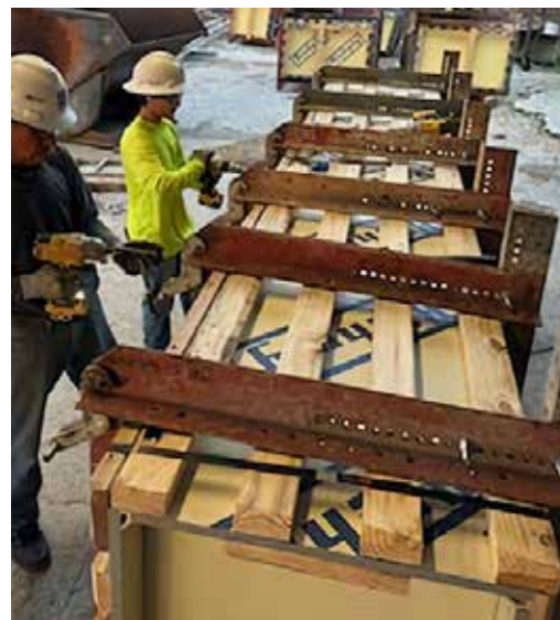
Fig. 2.6.7: Workers engaged in the assembly (make-up) of a column form. (Image courtesy of Ceko Concrete Construction.)
