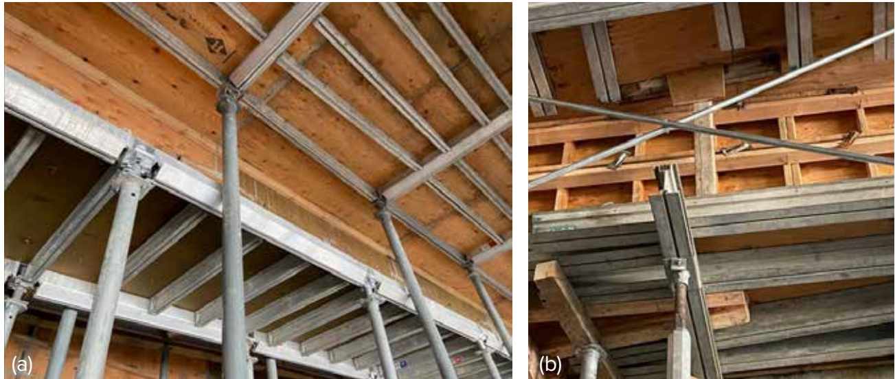
2.6.19: Photos of forms with beam sides connecting beam bottoms with slab soffits: (a) form depths of 20 in. or less allow form sides to carry concrete pressures with minimal members (photo courtesy of Ceco); and (b) form depths exceeding 20 in. necessitate studs, wales, and tie rods. (Image courtesy of Hensel Phelps.)
