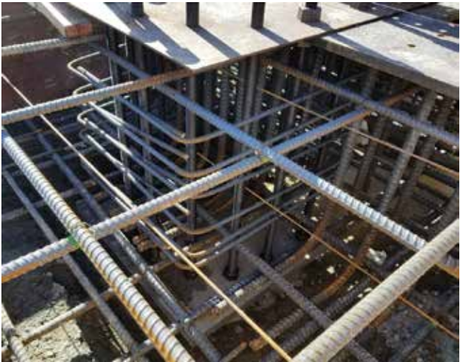
Fig. 2.12.4: Anchor bolts are positioned in a foundation element using a reusable alignment template. (Image courtesy of The Conco Companies.)
