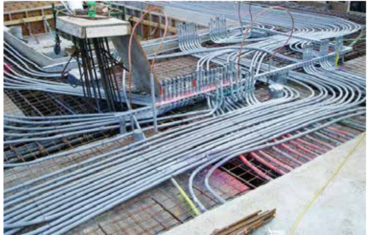
Fig. 2.7.41: This heavy concentration of electrical conduit conflicts with vertical reinforcement and will make it almost impossible for concrete to flow between the conduit and the forms below. (Image courtesy of Ceco Concrete Construction..)
