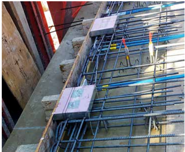
Fig. 2.7.42: Cladding connection systems are not all typical and should be considered for constructability in the reinforcing design as they may reduce clearance or displace reinforcement. (Image courtesy of CKC.)
