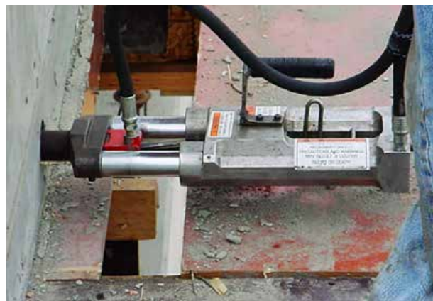
Fig. 2.7.36: The jacks used for tensioning PT cables require a 3 ft wide accessible zone. (Image courtesy of Post-Tensioning Institute.)
