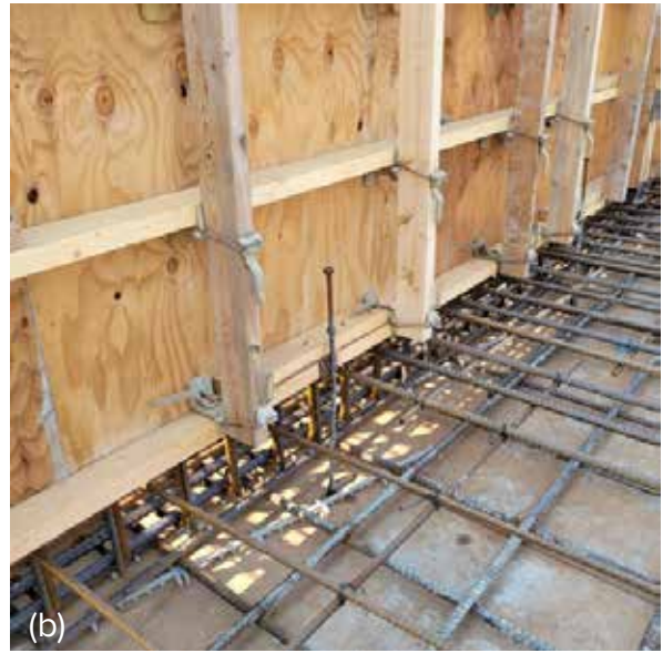
Fig. 2.6.31: Examples of problematic slab transitions: (a) the forms at this transition are not braced, increasing the risk of displacement during the concrete placement; and (b) this large transition will create high uplift pressures in the lower concrete surface, making it difficult to achieve the required surface finish. (Images courtesy of Ceco Concrete Construction.)
