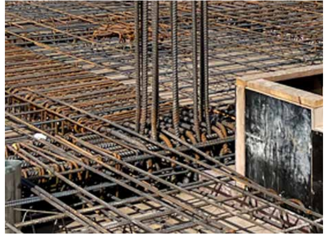
Fig. 2.7.20: Reinforcing bars at a beam-slab-column connection (photo courtesy of Ceko Concrete Construction.) Note that ACI 318 Section 24.3.4 requires tension reinforcement in beam and girder flanges (top bars at column intersections) to be distributed within the lesser of the effective flange width b_f or a width equal to 10% of the clear span l_n of the flexural member (refer to Fig. 2.7.27).
