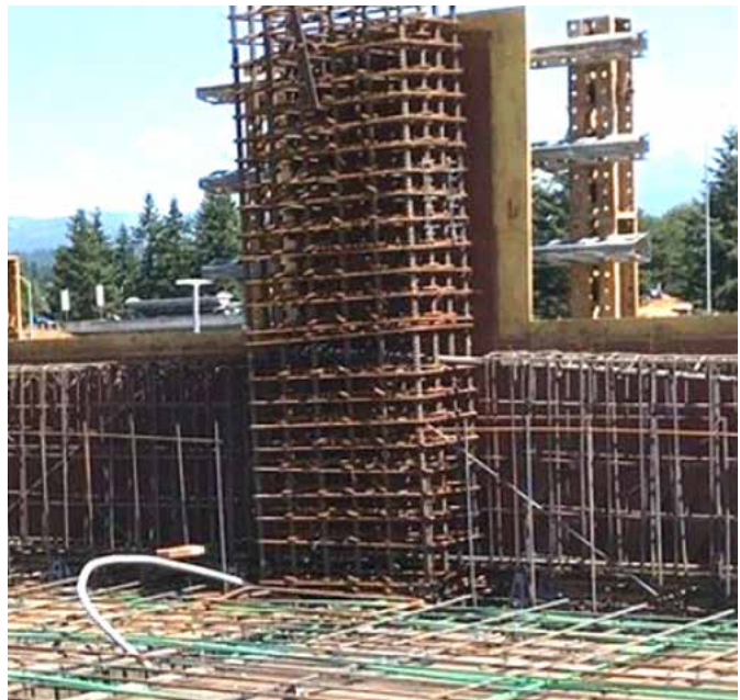
Fig. 2.11.2 Beam-column connections in rigid frames may present constructability challenges (photo courtesy of The Conco Companies).
