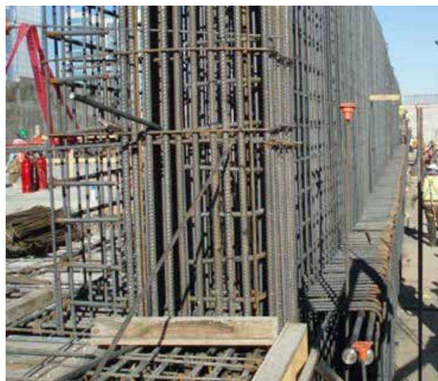
Fig. 2.6.39: Reinforcement and formwork placement for a deep transfer girder. The wide reinforcing cage below was designed as the reinforcing cage for a beam that will support the transfer girder and its formwork during placement, thus avoiding the need for shoring to support the full weight of the deep girder. (Image courtesy of Ceco Concrete Construction.)
