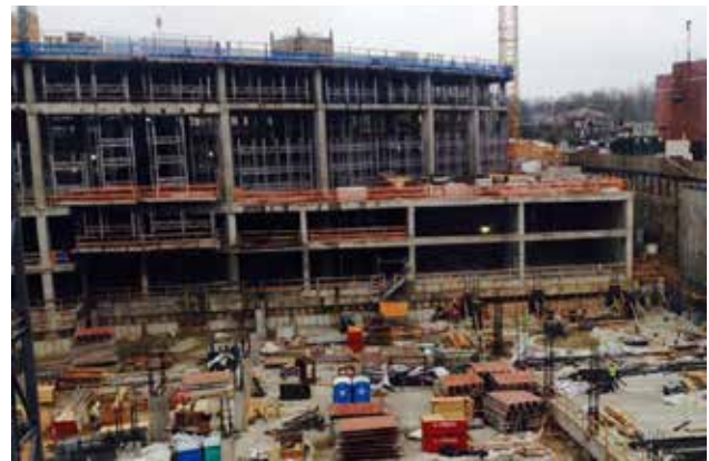
Fig. 2.6.15: A project with a tower structure isolated from a base structure. The separation followed a straight column line rather than the radius of the tower. (Image courtesy of Ceco Concrete Construction.)
