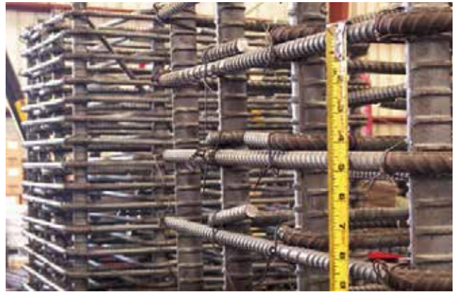
Fig. 2.7.10: Column cage mockups designed and fabricated using different grades of bars. The cage comprising HSRBs (foreground) required significantly less labor for bar placement and will allow much better flow of concrete between bars than would be required in a cage comprising Grade 60 bars (background). (Image courtesy of KKC.)
