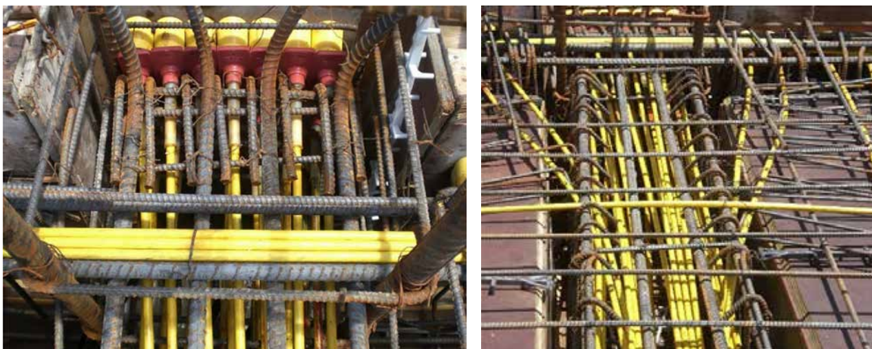
Fig. 2.7.45: Congestion in anchorage zones may prevent concrete consolidation. (Images courtesy of PTI.) Stacked and abutted PT tendon anchors indicate the beam width is insufficient for constructability. The most preferable solution would be widening the beam. Additional solutions could include flaring more cables, eliminating embedded items and MEP items in the congested zone, using headed bars or stud rails in lieu of hooked bars, or even using a multi-strand bonded PT system in the beam.
