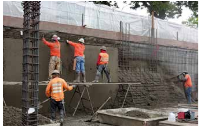
Fig. 2.12.10: Shotcrete operations require no formwork or tie rods. (Image courtesy of The Conco Companies.) Reinforcing bar congestion hinders shotcrete's applicability, especially at pilasters. To improve constructability, upsize reinforcing steel and embed the pilaster into the wall as shown in Fig. 2.6.10 Plan A.
