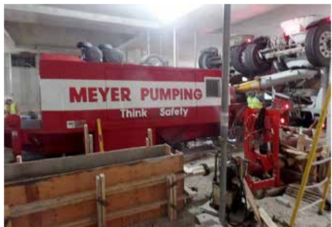
Fig. 2.9.9: A trailer pump positioned within a structure can convey concrete through a “standpipe” to the levels above. (Image courtesy of Ceko Concrete Construction.)
