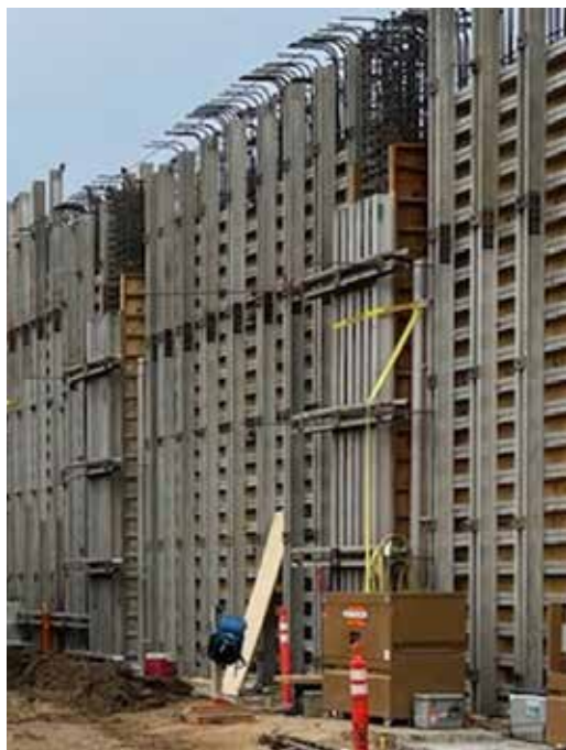
Fig. 2.6.9: Example of gang wall formwork with non-drafted pilasters. (Image courtesy of Hensel Phelps.)
