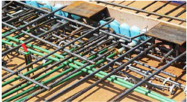
Fig. 2.7.43: Structural designers must coordinate embedded plates, anchors, reinforcing bars and PT systems. (Image courtesy of Ceco Concrete Construction.)
