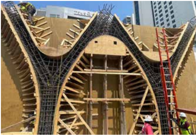
Fig. 2.6.16: An extreme example of an unusual and expensive column shape. Such features should be limited to structures in which such architectural statements are desired. (Image courtesy of Ceco Concrete Construction.)
