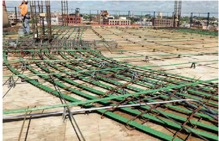
Fig. 2.7.51: Tendon sweeps should be anchored with hairpins if tendons are near slab openings and sleeves. (Diagram and image courtesy of Amsysco.)
