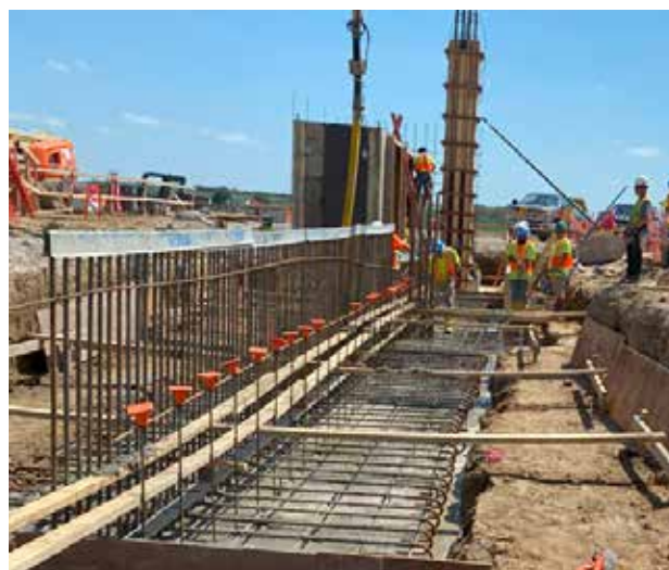
Fig. 2.12.2: Photos of continuous footings that have been prepared for bank pours. (Image courtesy of Ceco Concrete Construction.)
