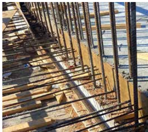
Fig. 2.6.11: Details requiring formwork surfaces to be penetrated by PT strands and reinforcing bars will mandate labor-intensive removal of forms and consume formwork materials. While the shown penetrations are not on a gang form, they may have prevented the use of such a productivity enhancing form system. (Image courtesy of Ceko Concrete Construction.)
