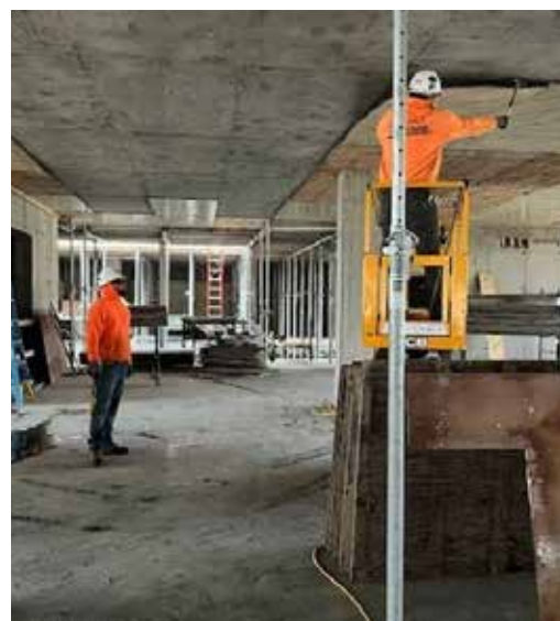
Fig. 2.6.12: Workers remove deck formwork before installing reshores. (Image courtesy of Ceko Concrete Construction.)
