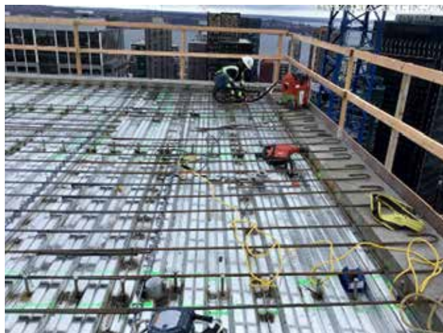
Fig. 2.11.4: Construction of a roof over an open shaft. This roof will comprise composite steel beams with a concrete slab on metal deck. (Image courtesy of The Conco Companies.)
