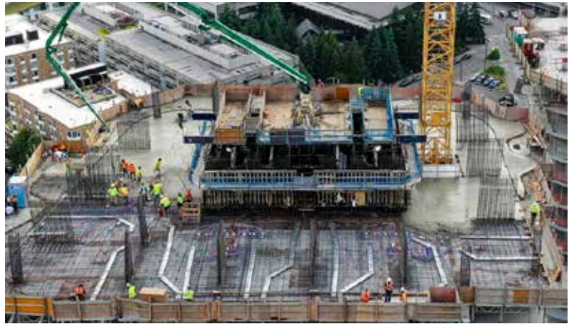
Fig. 2.7.6: Concrete placement on a floor structure. The structure will not be post-tensioned and the placement area is relatively small, so the contractor has elected to place concrete over the full floor area in a single pour. (Image courtesy of Ceko Concrete Construction.)
