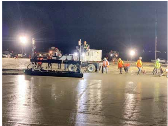
Fig. 2.7.5: A laser screed allows contractors to precisely strike off the concrete during slab-on-ground construction. (Image courtesy of Somero.)
