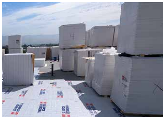
Fig. 2.9.11: Material will be stockpiled on decks, and these loads should be considered during design. (Image courtesy of Related.)
