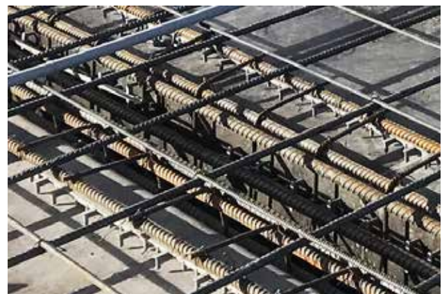
Fig. 2.7.22: Beam stirrups having out-turned hooks and open tops enable concrete placement and consolidation. Other constructable solutions include stirrups comprising baskets fabricated using welded-wire reinforcement. (Image courtesy of Ceko Concrete Construction.)
