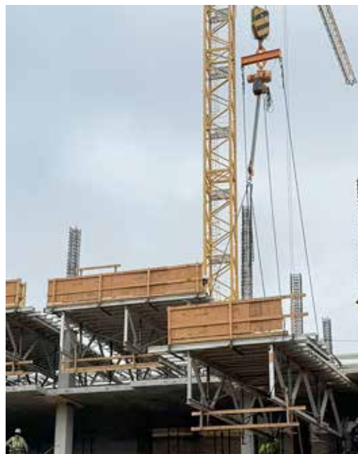
Fig. 2.9.1: A tower crane is used to lift a slab form. The center of such a load can be 30 or 40 ft beyond the face of the building. (Image courtesy of Hensel Phelps.)
