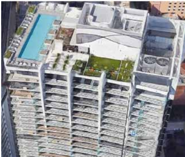
Fig. 2.6.44: A roof structure with a swimming pool, green roof, and mechanical equipment. High dead loads such as these may require a heavy structure that must be supported by multiple levels of reshores. (Image courtesy of Ceko Concrete Construction.)
