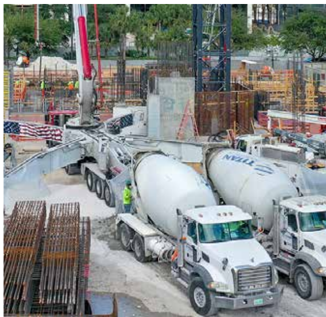
Fig. 2.9.6: A concrete pump on a tight site accommodating two mixer trucks. (Image courtesy of Ceko Concrete Construction.)
