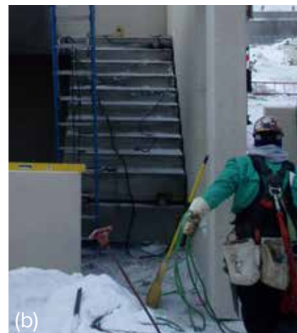
Fig. 2.6.25: Construction of concrete stairs: (a) cast-in-place concrete; and (b) precast concrete. (Image courtesy of Ceco Concrete Construction.)
