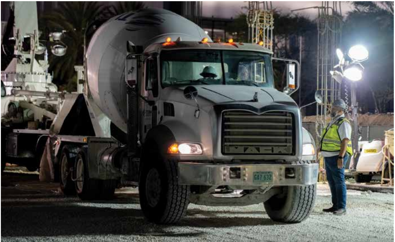
Miami World Tower. Image courtesy of Ceko Concrete Construction.
