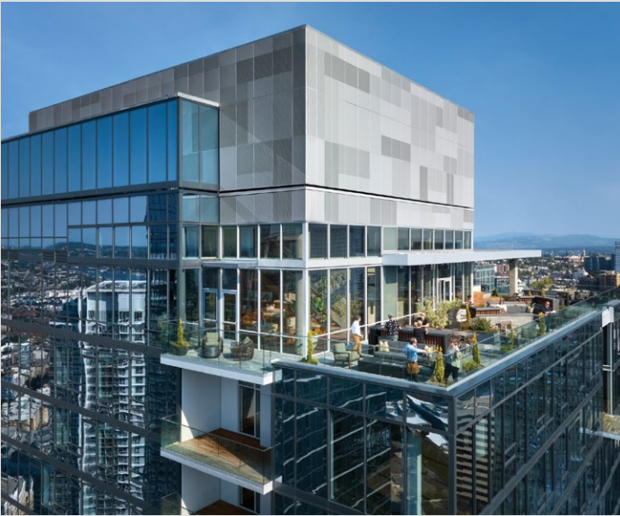
The Ayer's rooftop features floor-to-ceiling glazing and an expansive terrace, blending indoor comfort with sweeping skyline views.
