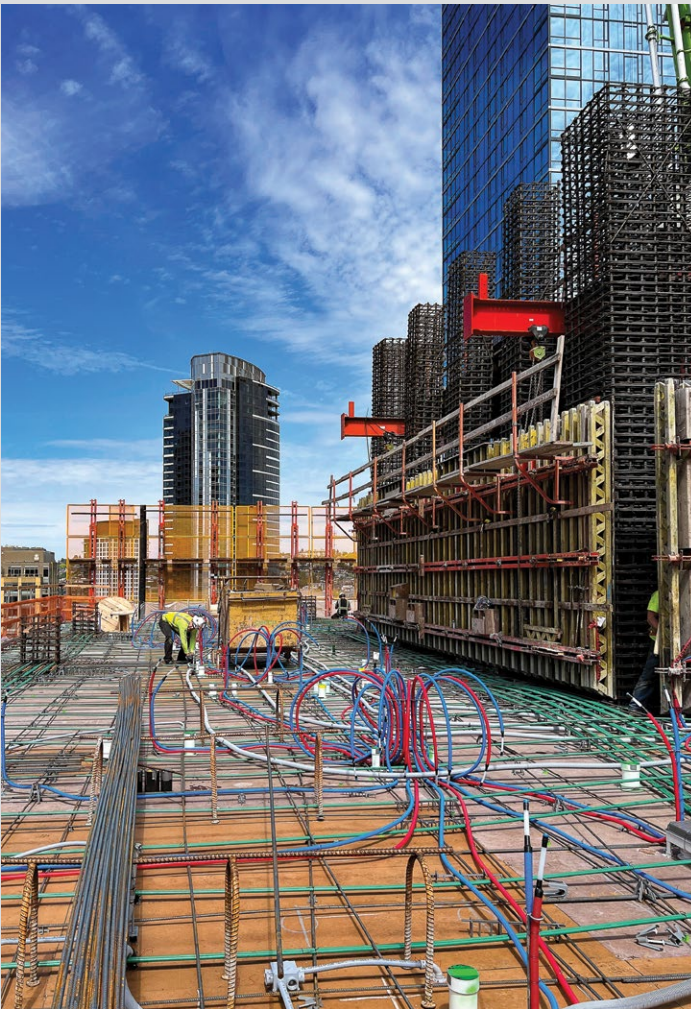
Slabs were post-tensioned and used perimeter cantilevers to improve efficiency.
