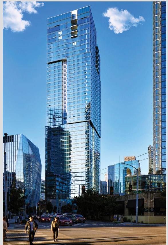
The Ayer is an iconic addition to downtown Seattle and used sustainability-enhancing Type 1L Portland Cement throughout, significantly lowering the building's embodied carbon footprint.
